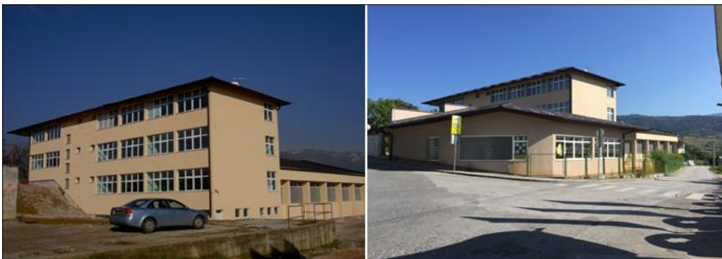
Left: Photo before the construction of the extended stay building and the arrangement of the amphitheater
