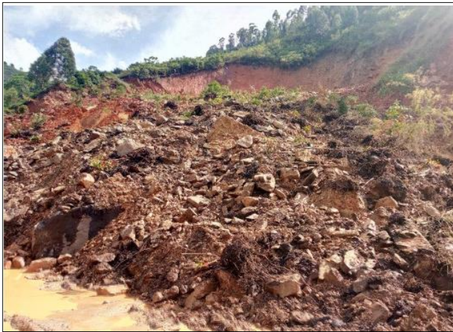
Fig 7: Landslide at makengele on the Goma-Bukavu road
