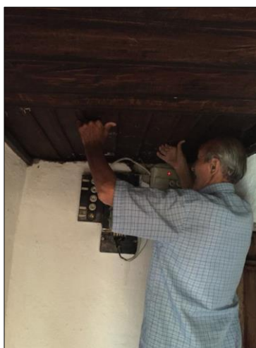
Fig 28: Cover in the ceiling floor-roof for exit to the roof space (left)
