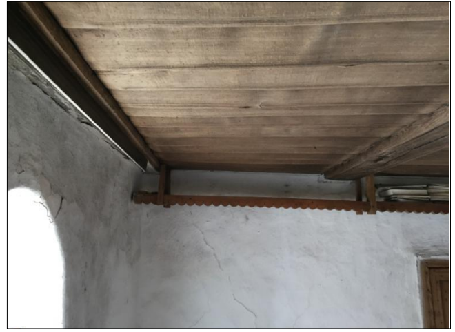
Fig 8: Wooden ceiling ('shishe') and shelf ('rafa') of the main room on the ground floor (left)
