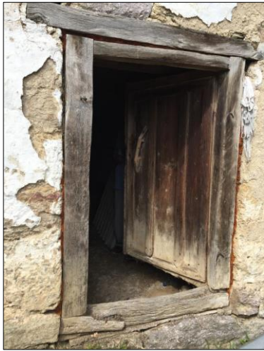
Fig 17: Basement door (left)
