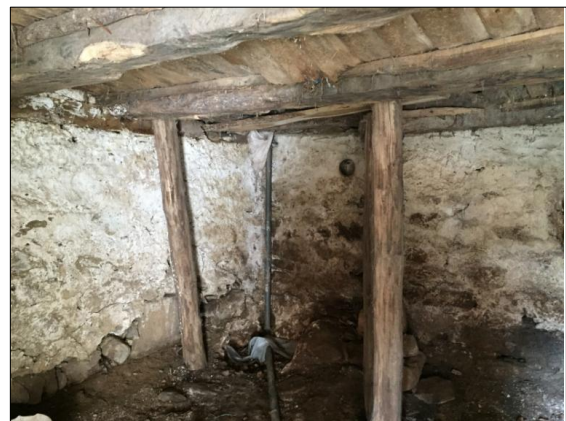
Fig 4: Basement interior (left)
