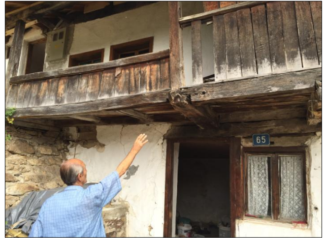
Fig 14: Place of exit of the wooden part of the staircase ground floor-first floor on the (original) divanhana and subsequent extension of the divanhana-veranda (left)
