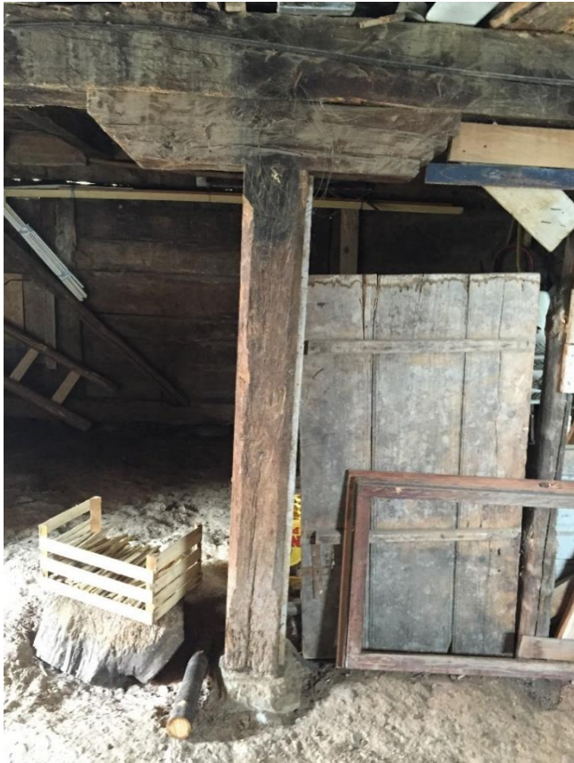
Fig 11: The Kasumovic family house in Vrnoegrac. The ground floor is arranged as a stable. A column in the middle of the barn is a typical solution in the Krajina chardaklija house
