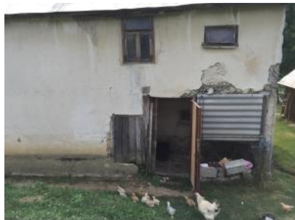
Fig 26: The Kajtazovic family house in the Donja Lucka settlement near Cazin. Left: view of the house from the northwest. Right: the once open space under the staircase was later fenced off and converted into a storage room and poultry house Source: Author (July 25,2016)
