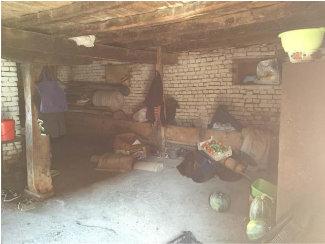
Fig 20: Former barn (ground floor), now large pantry
