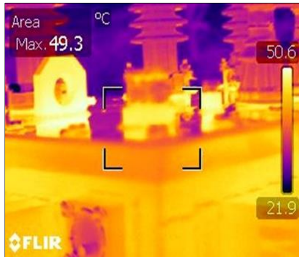
Fig 4: Transformer Top Packing Thermal
