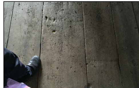
Fig 15: The Kovacevic family house in Vrazici near Celic. Massive wooden floors in the floor of one part of the 'kuca' ('mutvak')
