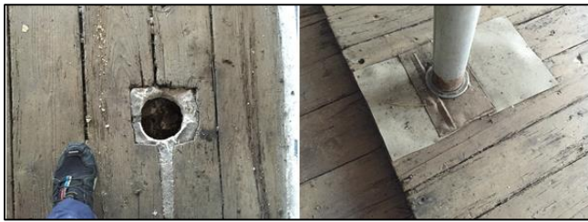
Fig 22: The Kovacevic family house in Vrazici near Celic. The place of penetration of the flue duct in the ceiling structure of the ground floor-floor
