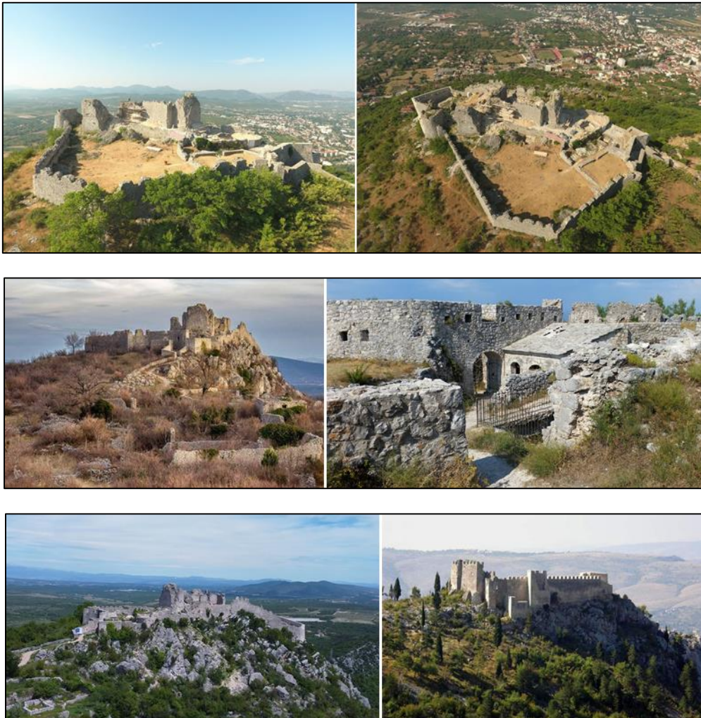
Fig 15: Tower of Herceg Stjepan Vukčić Kosaca in the Old Town Ljubuski http://ljubusaci.com/2021/09/12/tvrđava-hercega-stjepana-u-ljubuskom/ https://www.ljportal.com/price-mostar-hercegovinu-stari-grad-ljubuski-10844/ https://lh5.googleusercontent.com/p/AF1QipP7QtUbrarFH77SoX0KdBy2gcCT3n0ekRIeD-8X=h720 , Accessed: 11.22.2022. https://www.youtube.com/watch?v=8HIXIfGsEyc https://herzegovina.in/videostari-grad-ljubuski-uskoro-u-novom-ruhu/
