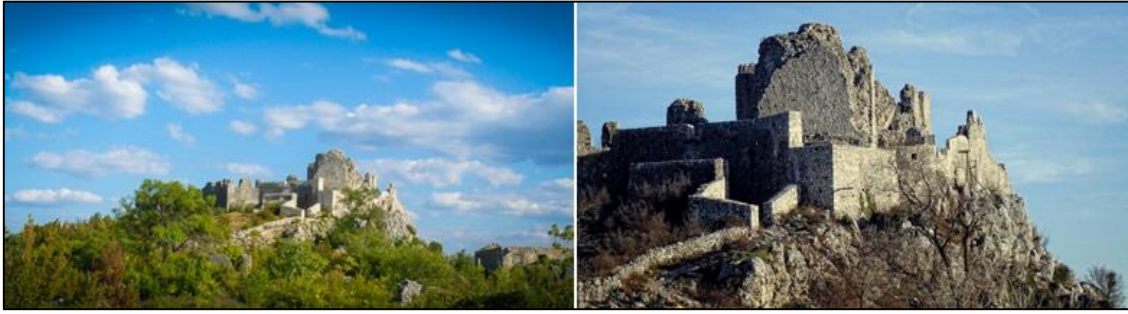
Fig 14: Tower of Herceg Stjepan Vukčić Kosaca in the Old Town Ljubuski http://herzegovina.travel/blog/listings/stari-grad-ljubuski/ http://nasatv.ba/pripema-se-dokumentacija-obnove-kule-ljubuskom/ http://medjugorje.info/medjugorje/index.php/hr/o-medjugorju/okolna-mjesta/ljubuski Accessed: 6.10.2018.
