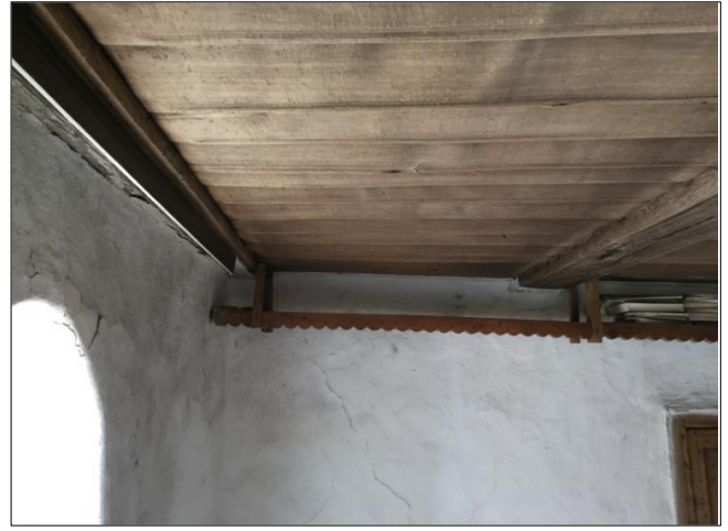
Fig 8: Wooden ceiling ('shishe') and shelf ('rafa') of the main room on the ground floor (left)
