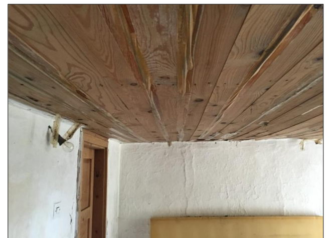
Fig 10: Wooden ceiling ('shishe') in the room created by the adaptation of the 'kuca' (left)
