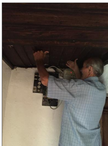
Fig 28: Cover in the ceiling floor-roof for exit to the roof space (left)
