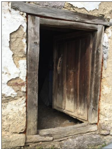
Fig 17: Basement door (left)
