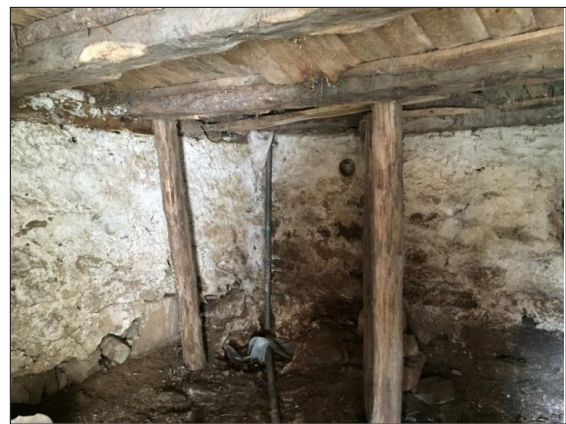
Fig 4: Basement interior (left)
