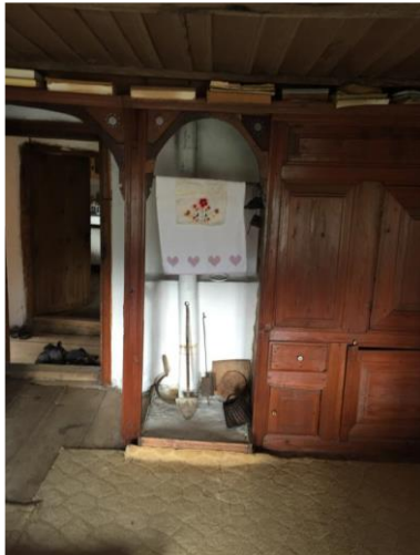
Fig 26: View from the main veranda towards the front door, hallway and living kitchen (left)
