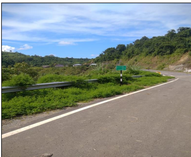
Fig 3: Kaladan Multi Modal Transit Transport Road at Zochachhuah, Mizoram
