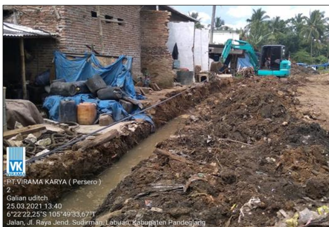
Fig 9: U-Ditch Drainage Work
