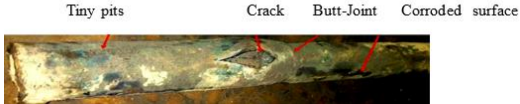
Fig 1: Sample of a failed portion of boiler pipe
