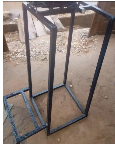
Fig 1: Constructed metallic support for the alternator
