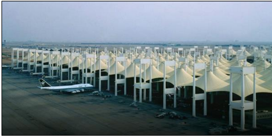
The existing terminal for pilgrims (The Hajj Terminal)
