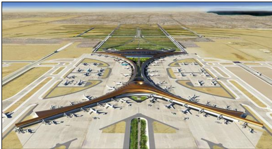
New airport (under construction)
