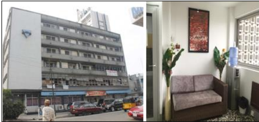
Fig 3: Exterior and interior YMCA building (source: etco-nigeria.com)
