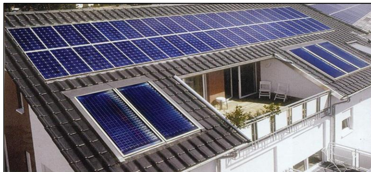
Fig 9: Photovoltaic panels integrated into building
