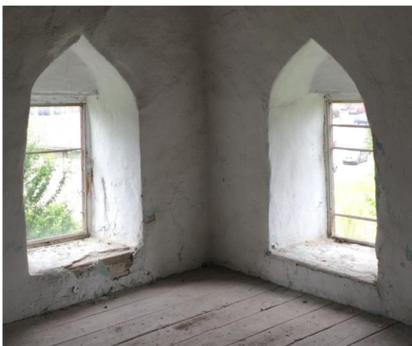
Fig 46: The house in Cuhovici near Konjic - window on a thick wall
