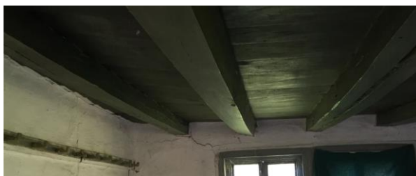
Fig 53: The Kovacevic family house in Vrazici near Celic - wooden ceiling in natural color and painted with green oil paint Source: Author (July 19, 2016)
