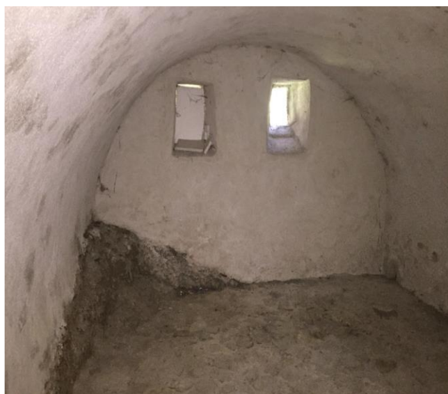
Fig 24: Krsnak's house 01 in Jajce. A stone vault as an inter-storey construction between ground floor and first floor Source: Author (July 21, 2016)
