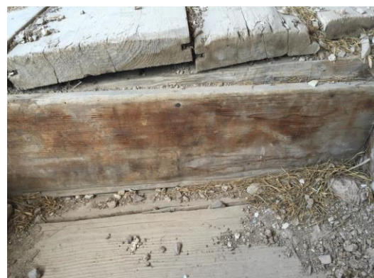
Fig 21: The Colak family house in the Brnjic village near Kakanj. The hewn wooden floors are about 7 cm thick
