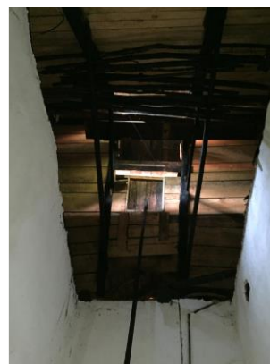
Fig 30: The Dusper family house in Kraljeva Sutjeska. Roof of the 'rafter with a crossbeam' type. Chimney with a strap for regulating ventilation
