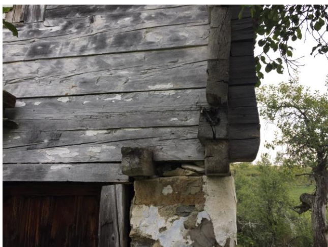
Fig 12: The house in the Visnjici village near Vares - building construction: ground floor walls made of hewn wooden logs
