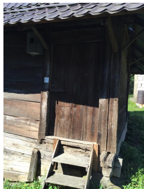
Fig 14: The Camdzic family house in Puracic near Lukavac - construction of the building: external walls of the ground floor (and basement) made of wooden logs Source: Author (August 4, 2016)
