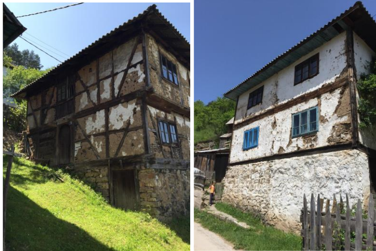
Fig 19: Left: the Smajic family house in the Starposle village near Kakanj - spatial-constructive structure of the building. The first floor is left to one side of the house. Right: Houses in the Brnjic village near Kakanj - the conceptualization and materialization of the walls clearly reflects their role in the constructive part of the building
