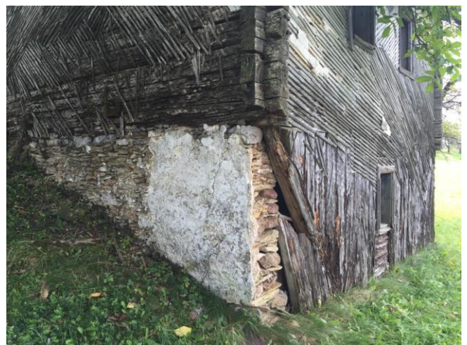
Fig 15: The house in the Dastansko village near Vares - structure of the building: basement walls made of stone and wooden 'ukobica', ground floor walls made of hewn wooden logs Source: Author (September 25, 2016)
