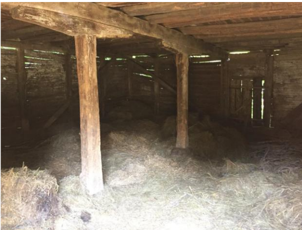
Fig 16: The Cekic family house in the Poljak neighborhood, Sanski Most: exterior walls of the ground floor made of wooden planks; massive wooden columns support the main wooden ceiling beam, which is supported on the column via a 'saddle'
