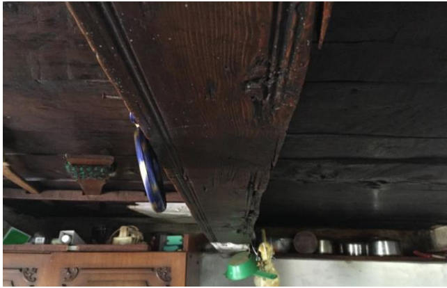
Fig 52: The Tresnjo family house in Cuhovici near Konjic - natural wood color in the smoke-impregnated wooden ceiling Source: Author (August 13, 2016)
