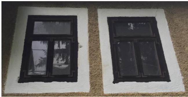
Fig 45: The House in Vrnogracki kriz at Velika Kladusa. Three-leaf windows, one wing of which is 'na ventus'
