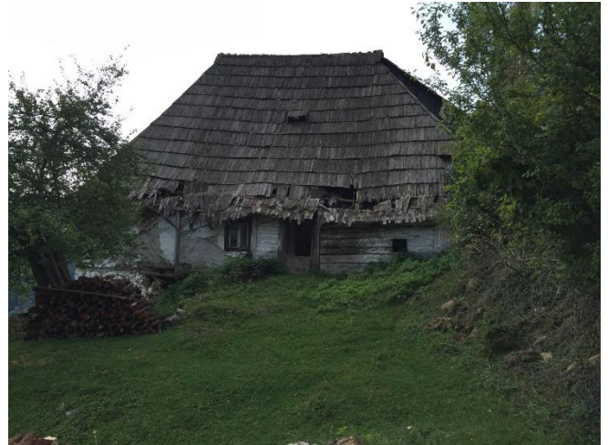
Fig 18: The Lekic and Mirkic families house in Przici near Vares - construction of the building: the exterior walls of the ground floor are made of wooden logs (and some of the wooden frame with a wooden frame)
