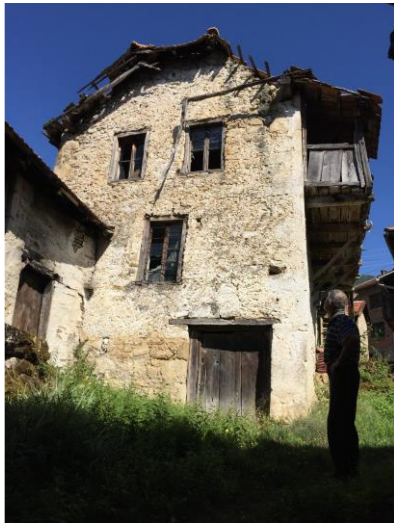
Fig 10: The houses in the Gorani village near Konjic - construction of the building: combined solution of the materialization of the walls
