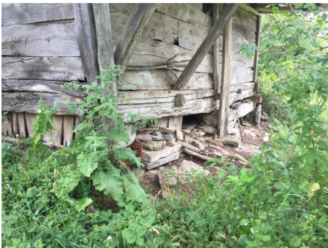
Fig 6: Individual foundation stones support the foundation beams and the entire structure of the house. The Abazovic family house in Donja Koprivna near Cazin
