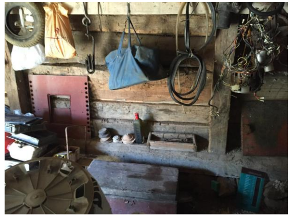
Fig 13: The house of the Ahmic family in the Brizdje village near Zepce - wooden basement walls in contact with the ground Source: Author (July 18, 2016)
