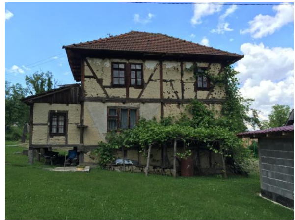
Fig 57: Left: The Camdzic family house in Puracic near Lukavac - contrast of the dark, natural color of the wood and the white painted surfaces of the walls of the ground floor and first floor.
