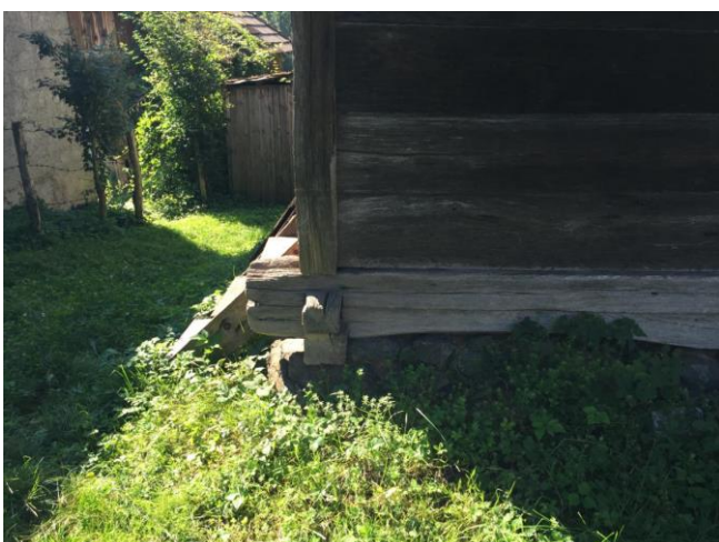
Fig 7: The Camdzic family house in Puracic near Lukavac - wooden foundation beam placed on a series of foundation stones
