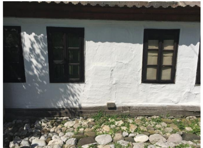
Fig 8: The Smajlovic family house in Cehaje near Srebrenik - wooden foundation beam placed on a series of foundation stones
