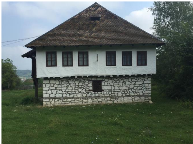
Fig 17: The Korajlic family house in Hrvatinovici near Tesanj - construction of the building: ground floor walls made of finely worked stone
