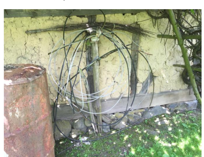
Fig 9: The Ejubovic family house in the Poljice village near Lukavac - wooden foundation beam placed on a row of foundation stones.
