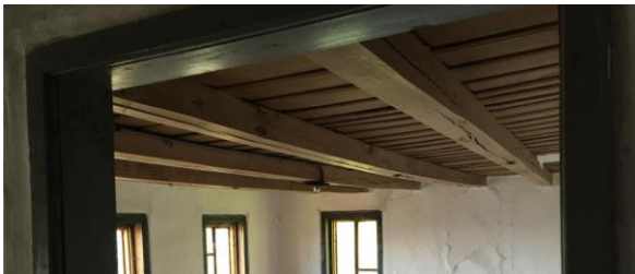
Fig 52: The Tresnjo family house in Cuhovici near Konjic - natural wood color in the smoke-impregnated wooden ceiling Source: Author (August 13, 2016)
