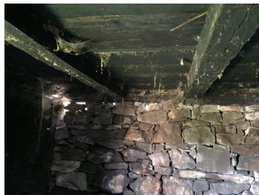
Fig 49: Stone wall (towards the ground) and wooden ceiling (impregnated with smoke) in the Smajic family house in the Starposle village near Kakanj
