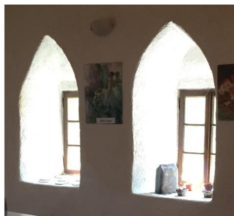
Fig 47: Left: the Pozderac family house in Cazin - windows in thick walls. Right: Musafirhane in Fojnica - window in thick wall of ground floor
