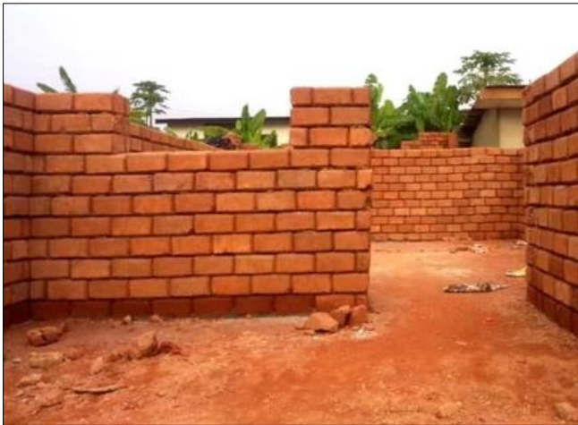
Fig 5: Showing Erection of Walling Units
