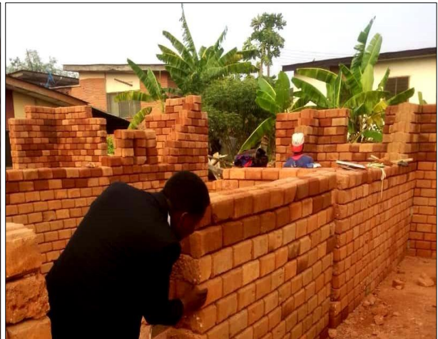
Fig 5: Showing Erection of Walling Units
