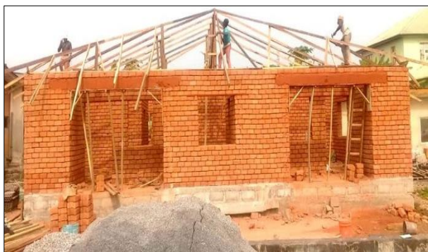
Fig 6: Lintel Installation
