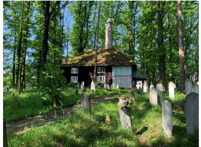
Mosque built from oak logs taken on site
