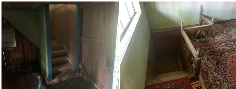
Wooden stairs from the ground floor to the gallery ('mahfil') made of carved oak beams
