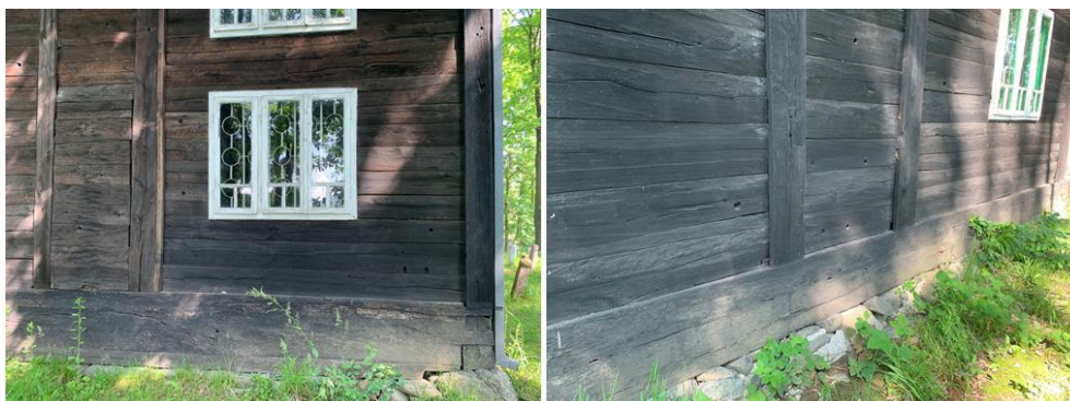
Detail of the mosque's construction: stone foundations and walls made of hewn oak logs
