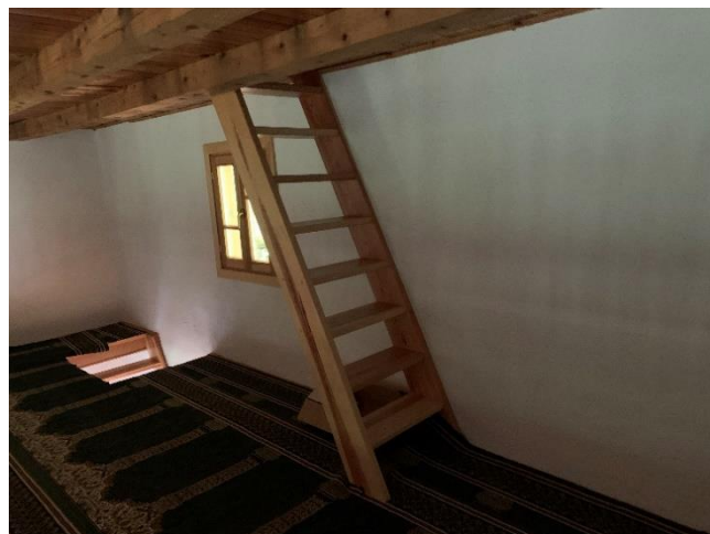
Wooden staircase ('basamaci') for the exit to the attic space from the gallery
