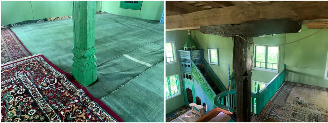
Left: The central pillar supporting the gallery ('mahfil') of the mosque. Right: The central pillar and main beam supporting the roof of the mosque. This pillar is in the same axis as the pillar in the landscape supporting the gallery ('mahfil')
