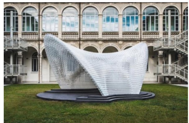
Fig 4: Trabeculae Pavilion 3D printed lattice structure at construction scale (Naboni, Kunic & Bressegello, 2020).
