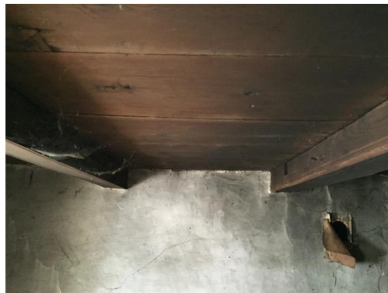
Fig 20: Interfloor structure ground floor-first floor, in a room, above the basement. The beams and floors are hewn. Over time, the wood has acquired the color of honey, and is impregnated with smoke that was let into the room from the space of the 'house'
