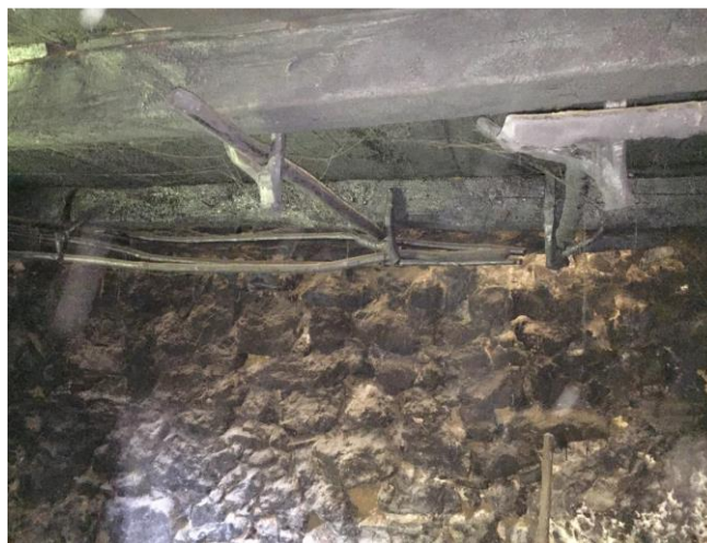
Fig 29: Wooden bars above the hearth on which kettles for cooking food are hung
