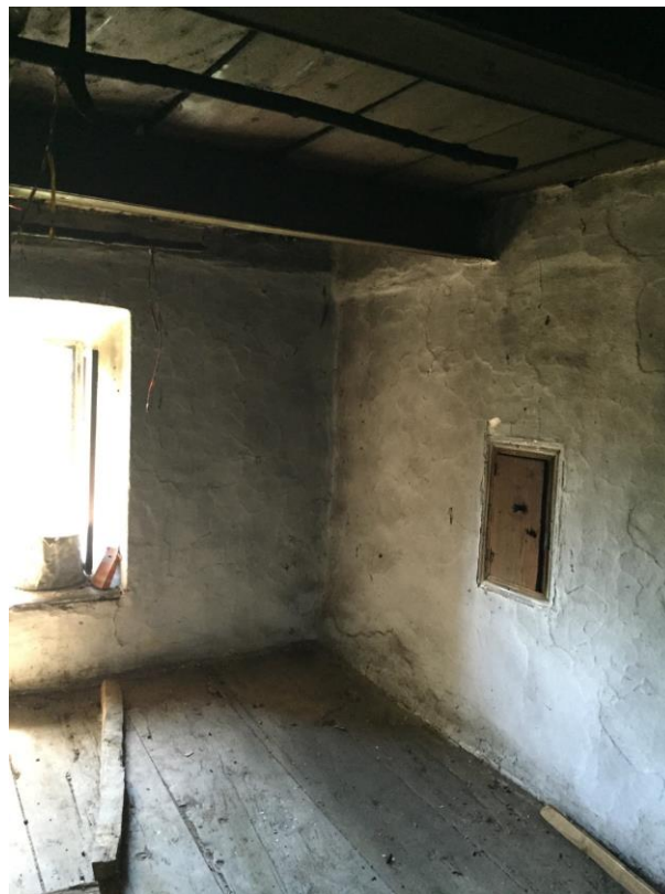
Fig 21: Surface treatment in the čardak area, above the room: wooden ceiling, a niche in a thick stone wall that is plastered and whitewashed, wooden floor...
