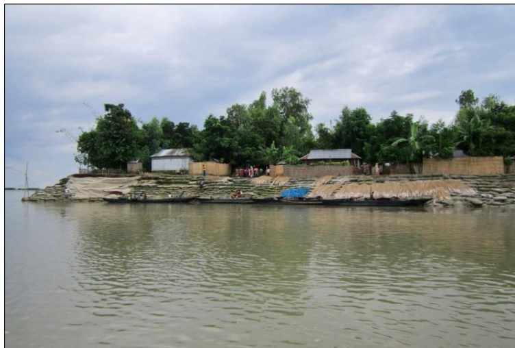
Fig 14: Bags of soil placed along the edge of charred land to prevent river erosion during monsoon floods
