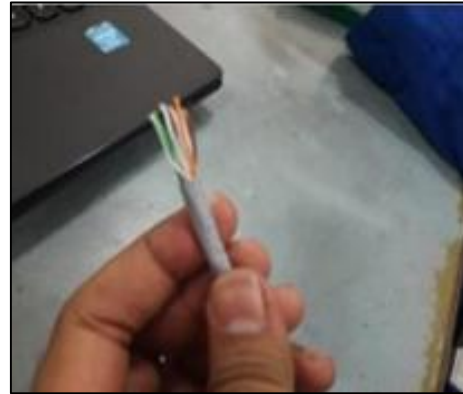
Fig 1: Peel the Protective Skin on the UTP Cable ( Situsnesia.com )
