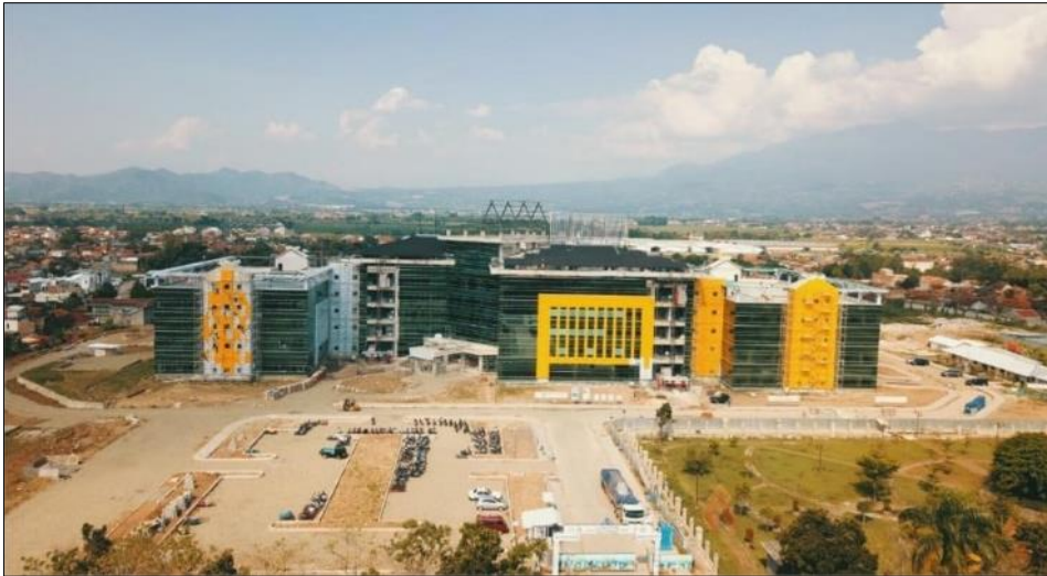
Fig 1: Soreang District Hospital Project on 20 July 2020
