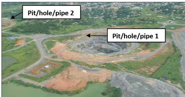
Fig 1: General View of The Koidu No.1 Pipe/Hole Vertical Pit
