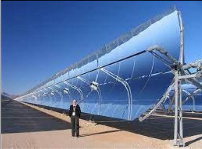
Fig 1: Parabolic CST system
